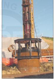
Bottom Drives for up to 36" upto 10' (3m) piles available including extended boots for batter/raked piles.
