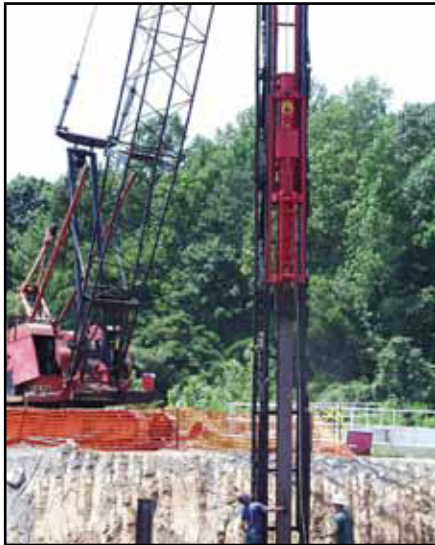
AD16-52 driving H-beam.
