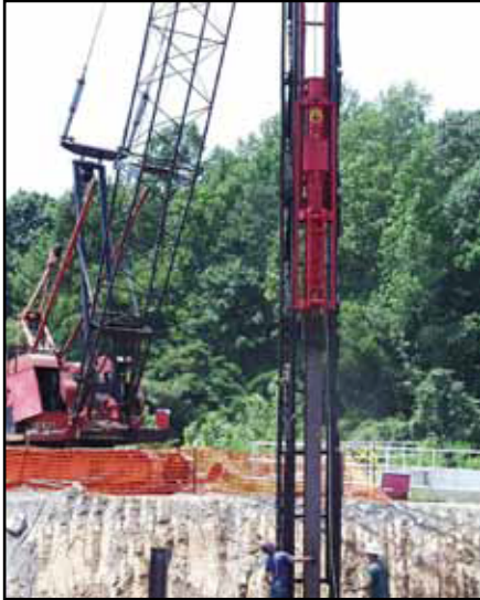
D19-52 driving H-beam.
