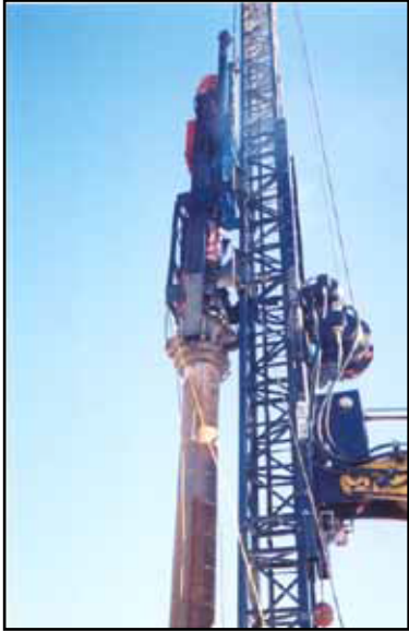
D25-52 with Excavator Mounted Leader.
