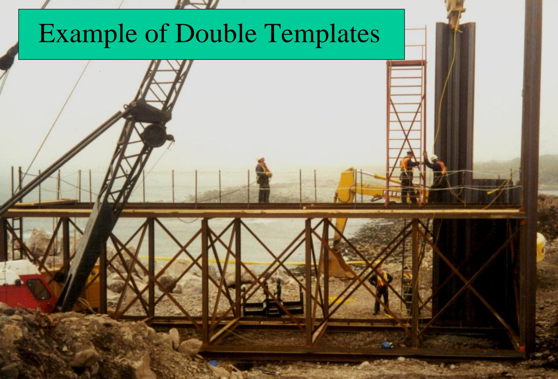
Upper template should be substantial fraction of the pile length.
