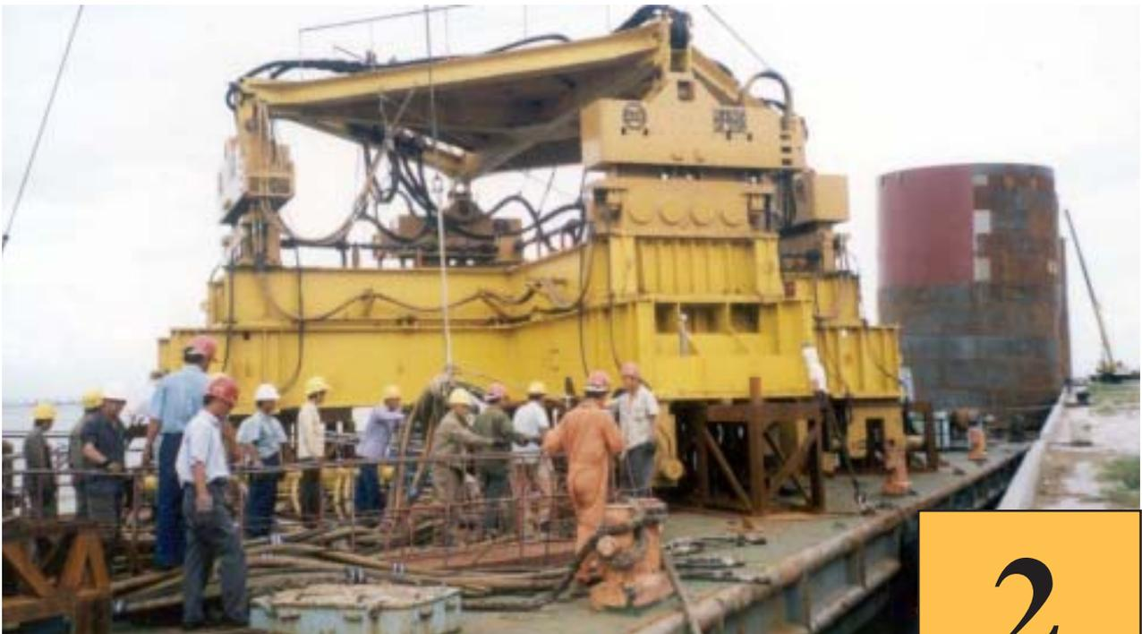
Quad 400 shown here with massive additional beam mounted under standard caisson beam to allow adaptation to larger 44 foot diameter steel piles.
