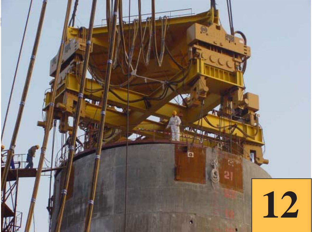
The first concrete pile was driven as fast as the crane operator could lower the block.
